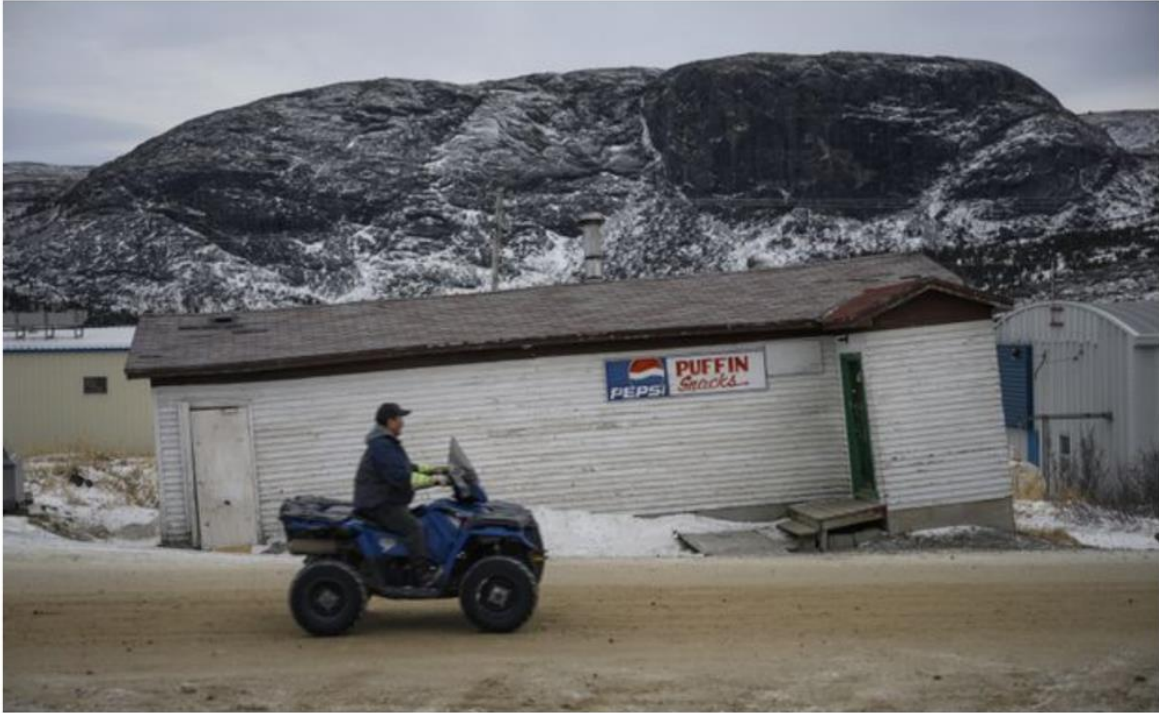
Figure 1.10. Sinking of a building due to thawing of permafrost [26].
