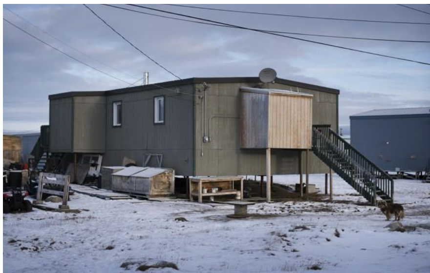
Figure 1.12. House in Clyde River, Nunavut raised on piles to avoid contact with frozen ground [45].
